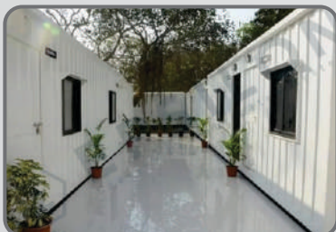
Site Office Containers
