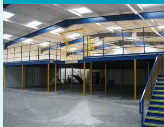
Mezzanine Floor View
