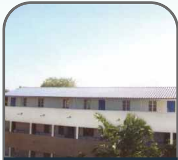
Roof Top Rooms
